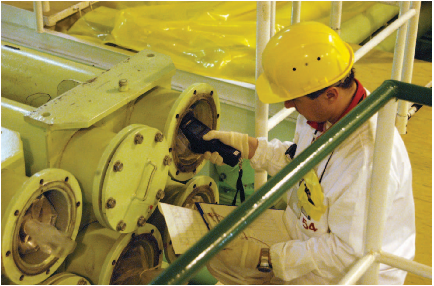
IAEA safeguard inspector checking fuel assembly in a transport container located in the fresh fuel storage of the Mochovce nuclear power plant. (IAEA Photo by Dean Calma)
