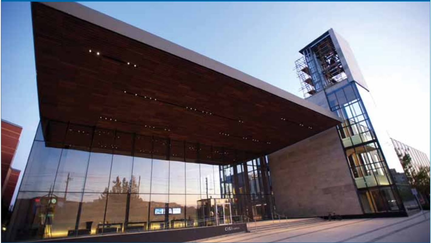
Construction of the 114,000-square-foot academic research complex on the CIGI Campus neared completion in fiscal 2010-11. The Campus is home to the Balsillie School of International Affairs. Possible future tenants include a proposed international law program, expected to be announced in early 2012.
