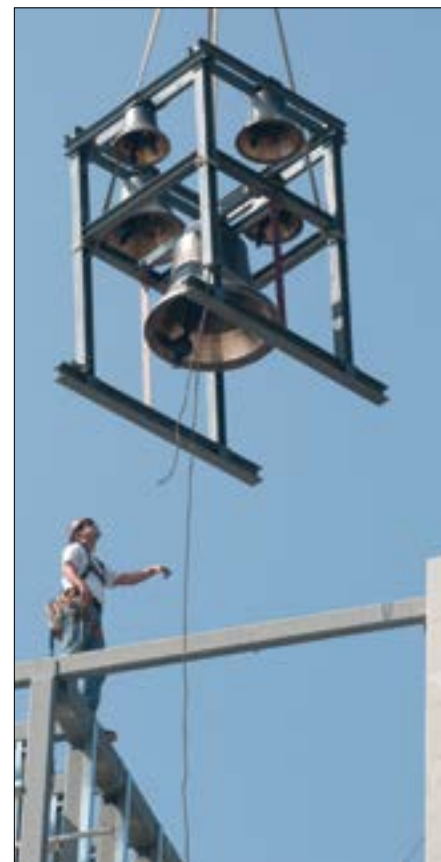
The bell assembly was raised up to the bell tower in August 2011. The five bronze bells were cast in Georgetown, Ohio.
